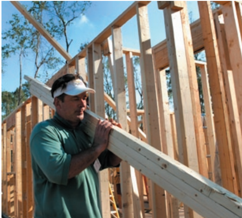
Courtesy of Habitat for Humanity
